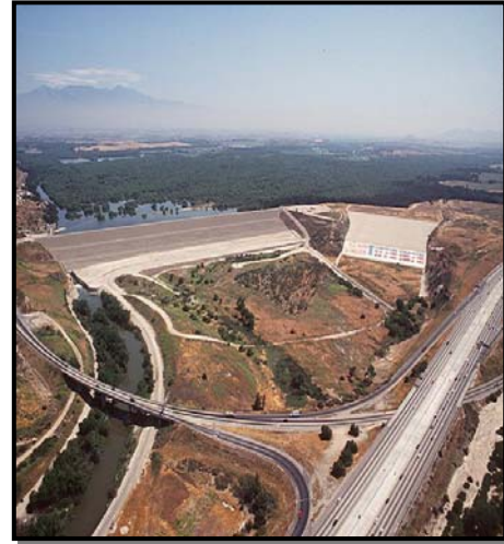
Prado Dam Source: United States Army Corp of Engineers Website
