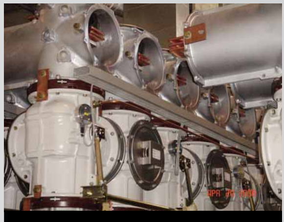
A portion of the 12-kV GIS switchgear being assembled.
