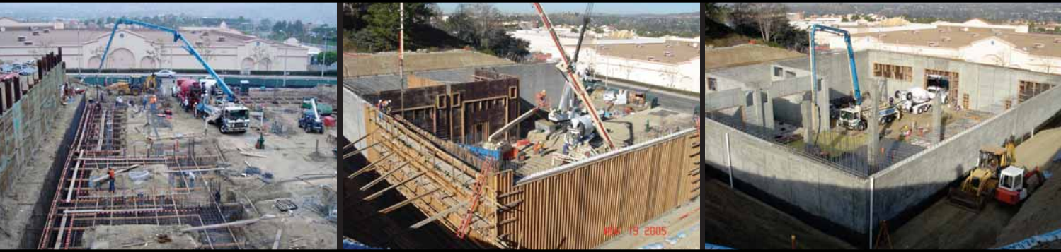
Construction sequence ending with a photo during dedication.
