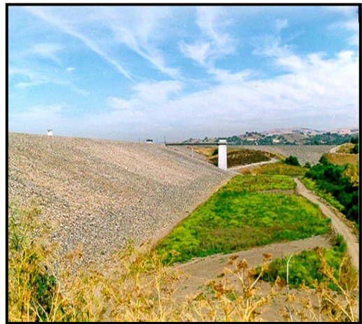
Carbon Canyon Dam Source: United States Army Corps of Engineers Website
