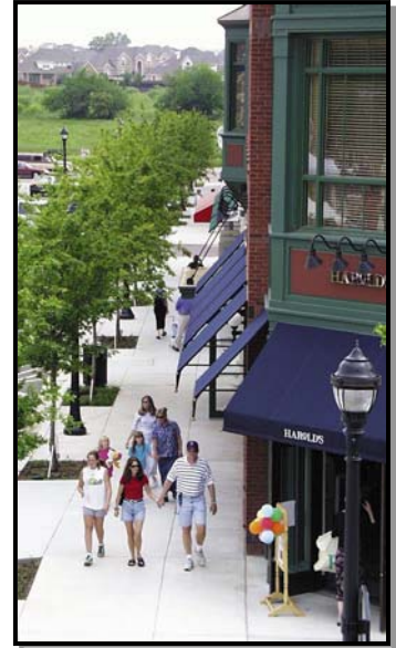
Siting buildings close to the street with visible entrances and pedestrian amenities invites use.
