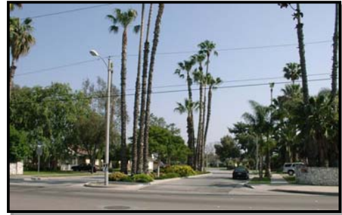
This neighborhood entryway at the intersection of Romneya and Euclid Street demonstrates that neighborhood identity can be improved with enhanced entry treatments – landscaped medians, distinct crosswalks and wide sidewalks.
