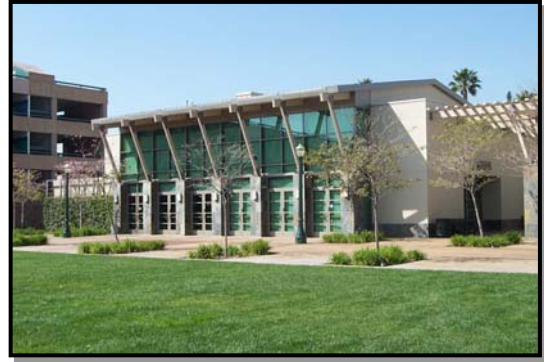
Anaheim's Downtown Community Center is an example of a modern building whose scale and detailing contribute to the character of the Downtown.
